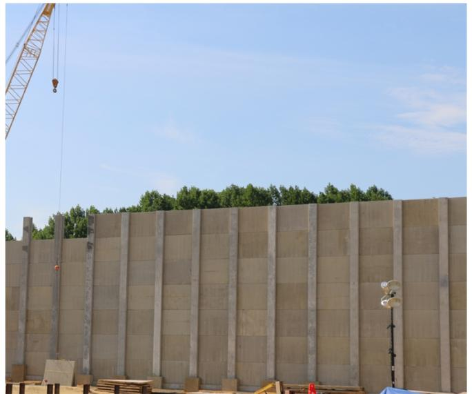
As of the end of July, about 400 cubic yards of concrete has been poured for the sound wall pedestals, 108 panels have been installed, and 67 precast posts and 16 sound wall grade beams have been set. The majority of the sound wall will be completed in the next few months.
